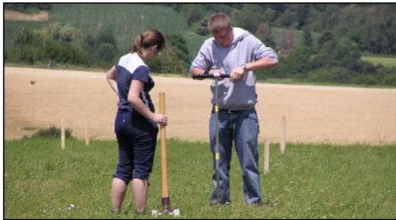
near-surface transmission lines
